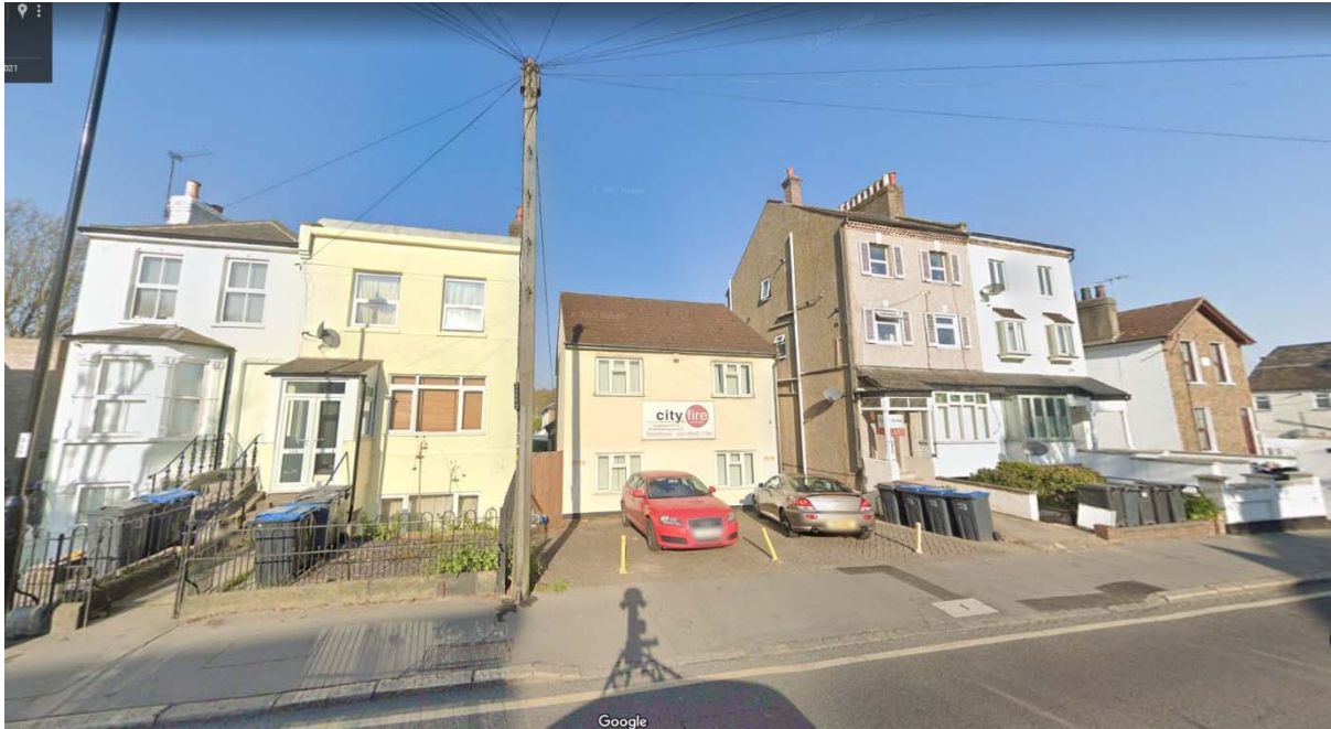
Figure 1 – front of site with adjoining premises
